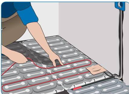
6) Install the Deviflex™ heating cable. Make sure that the cable, end termination and warm/cold cable connection are in contact with the aluminium plate or aluminium tape at all times.
